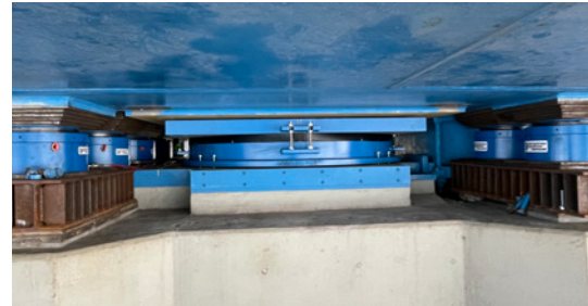
Installed new spherical bearing.
