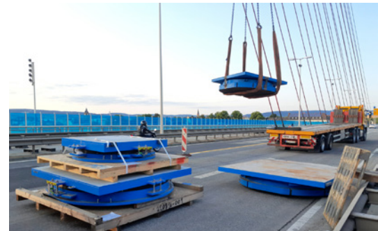
The new spherical bearings were replaced from the bridge deck.
