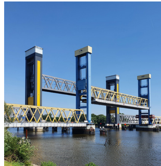
The Kattwyk bridges in the port of Hamburg: at the front, the new bridge for rail traffic, at the back the old bridge built in 1973, which now only carries road traffic.
