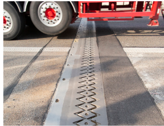
The new roadway expansion joint open for traffic. Photo: MAURER
