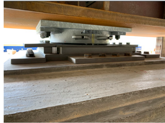
Installed bearing with steel girder laid on top.
