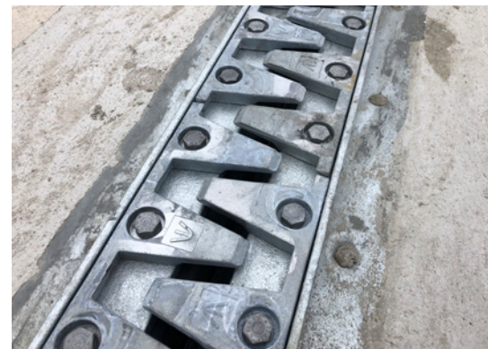
XC1 expansion joint embedded in concrete in Oosterhout in the south of the Netherlands. Visible at the upper side: the M-Plates.
