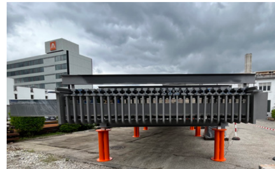
The massive expansion joint waits to be transported to China at the MAURER yard in Munich.
