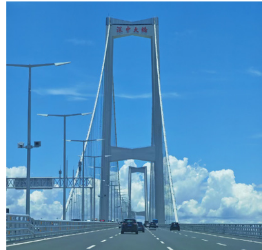
The main bridge of the Shenzhong Link, with its 1,666 m main span and bridge deck 91 m above the sea.
