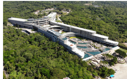
The Secrets & Dreams Bahia Mita hotel complex in Mexico was built step by step into the rising terrain and stands entirely on seismic isolators.
