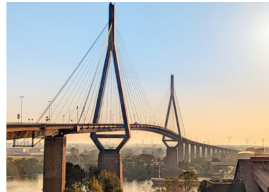
The Köhlbrand bridge in Hamburg.
