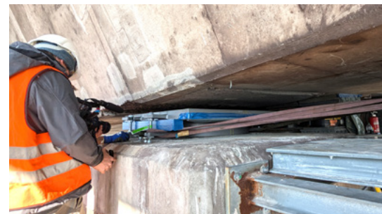
New inserted bearing.
