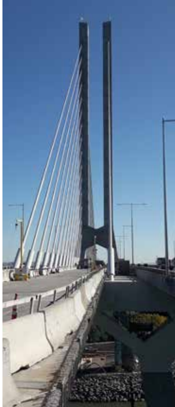
The 16 guided cross-ties were installed between November 2020 and April 2021.
