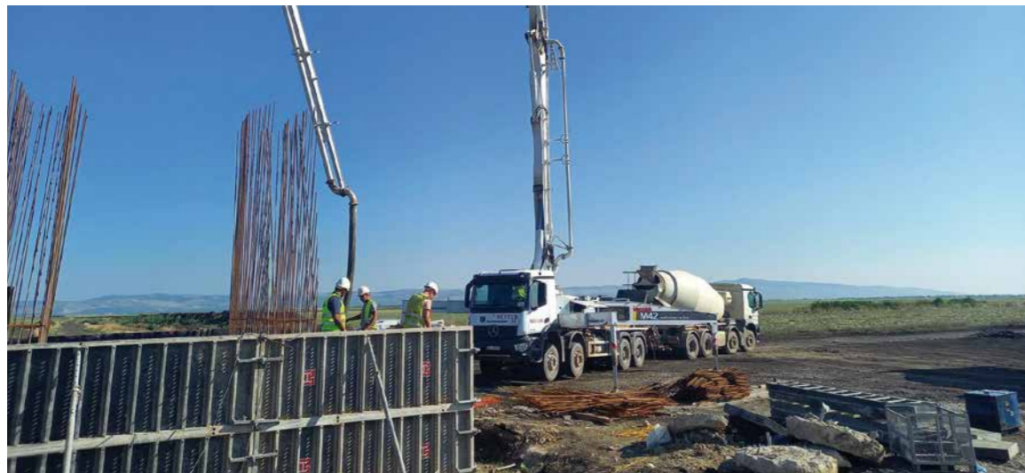
Motorway A0, several bridges with MAURER modular expansion joints.
