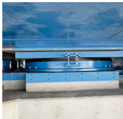
Installed new spherical bearing. Photo: MAURER
