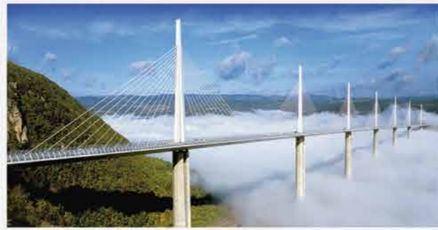
The Millau Viaduct carries the A75 motorway over the Tarn in southern France and, at 2,460 metres, is the longest cable-stayed bridge in the world.
