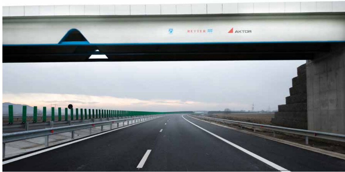
Motorway A7 Ploiesti-Buzau complete construction including several bridges with MAURER LRBs and modular expansion joints.
