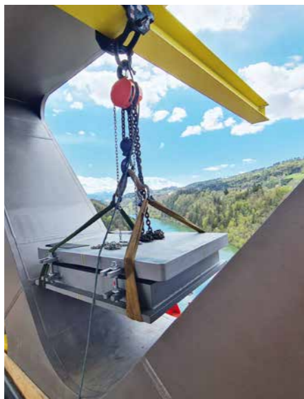
Lifting in the SIP® bearings using specific mounting girders. Photo: MAURER
