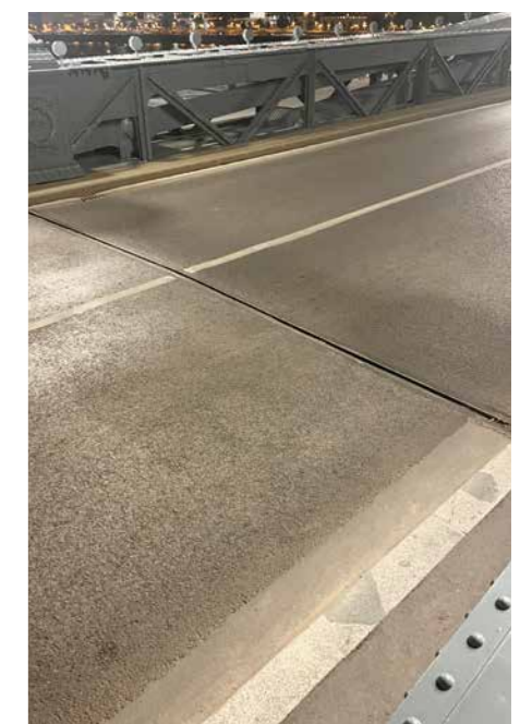
Installed expansion joint Photo: MAURER
