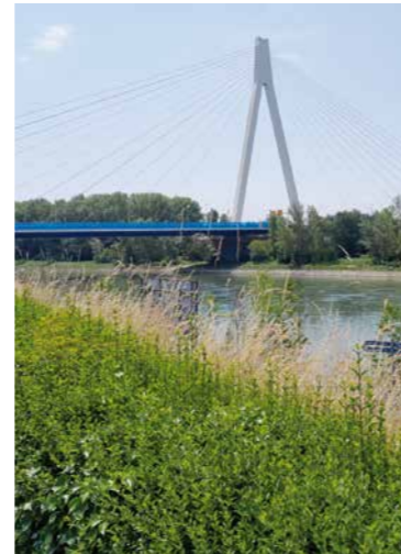
The Raiffeisen Bridge near Neuwied with the pylon on the Rhine island “Weißenthurmer Werth”. Photo: MAURER
