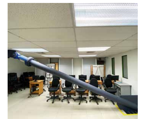
Built-in hydraulic damper: At the top with connection to the existing building structure. Photo: MAURER
