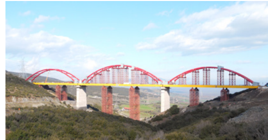
The SG26 is part of the new high-speed railroad line Tithorea-Domokos.
