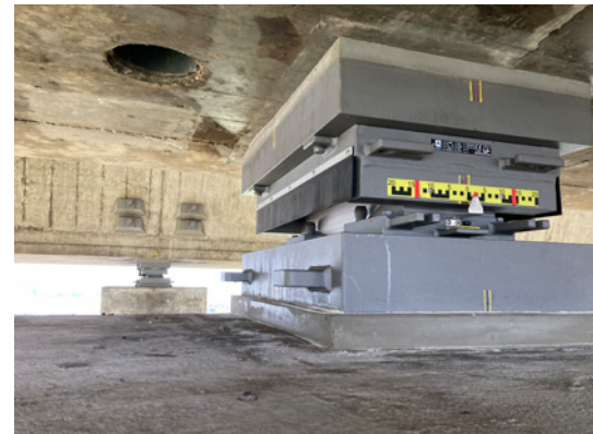
One of the 24 newly installed spherical segment bearings.
