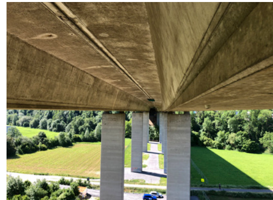
View below the bridge with the wide roller bearings.
