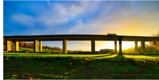
The Kocher Viaduct in backlight.
