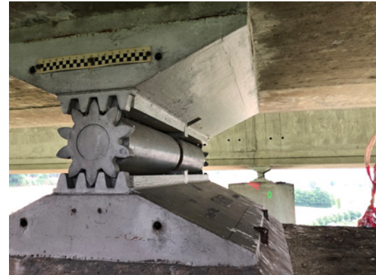
The old roller bearings prior to dismantling.
