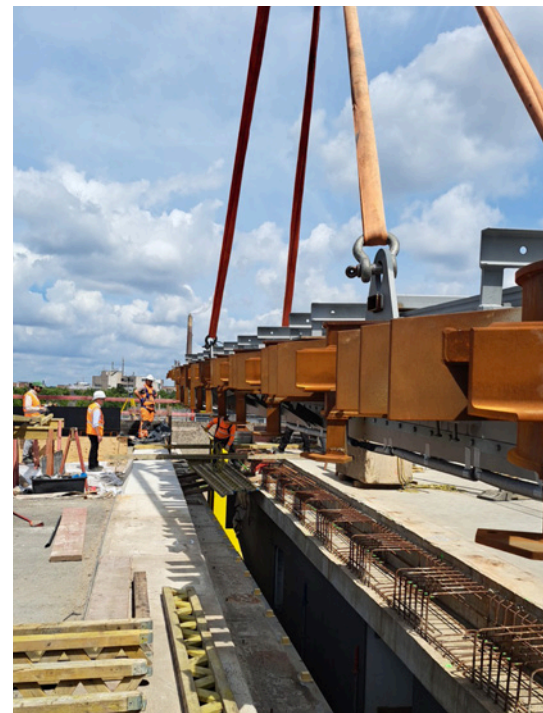
Lifting a large expansion joint into position in August 2023.
