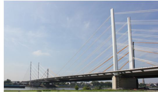
The Neuenkamp Rhine Bridge near Duisburg with completed southern superstructure (at the front).
