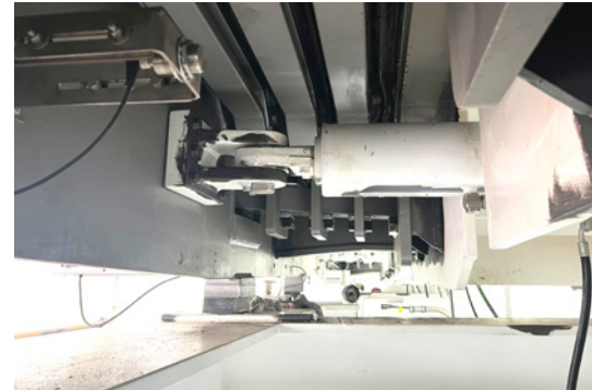
A look beneath the special construction. At the top are the grey intermediate beams. The hydraulic system is in the middle and behind it the swivel joists. The white area is the steel structure of the bridge.
