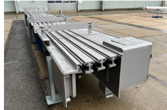
The special expansion joint prior to installation. The left side is welded onto the bridge. To the right of the intermediate beams is the 40-cm-wide piece that will rest against the northern half of the bridge.
