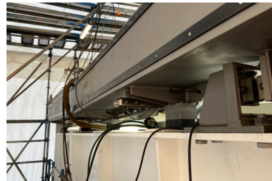
The fully cabled bridge during testing of the hydraulic functions.
