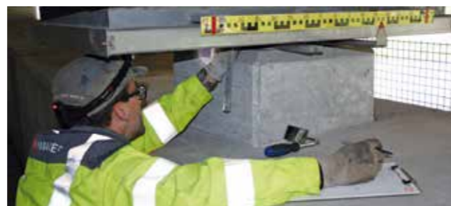
Inspection of bridge bearings
