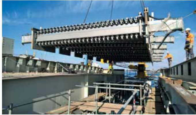
Installation of MAURER Modular Expansion Joint for Izmit Bay Bridge
