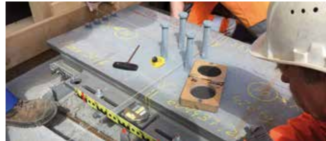
Installation Botlekbrug, Netherlands
