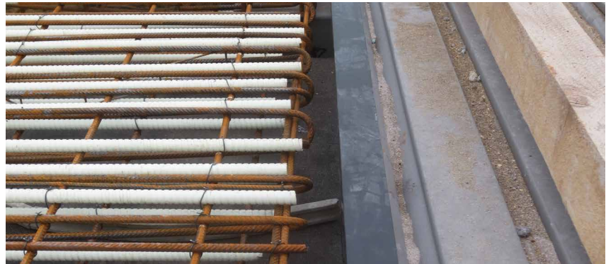
Clamped edge profile protection
