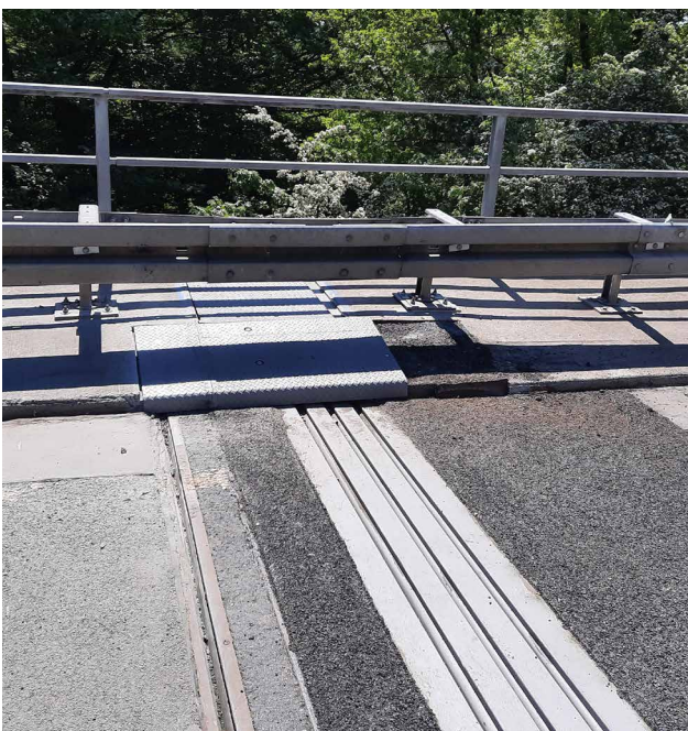
50 hours after the start of the construction site
