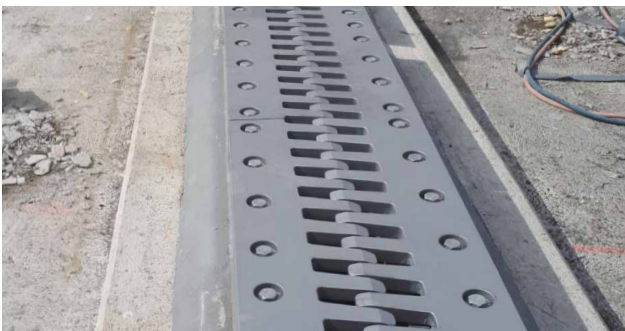
Bolted finger joint (FB)
