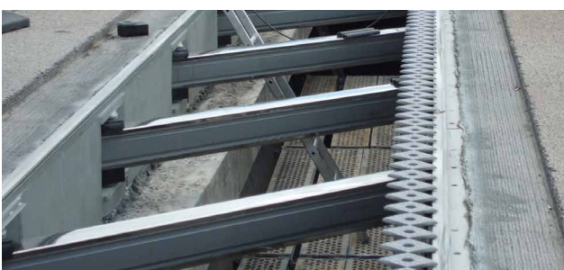
New support bars, refurbished edge structure
