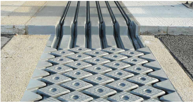
adjacent transition bar at XD6 using Betoflex®
