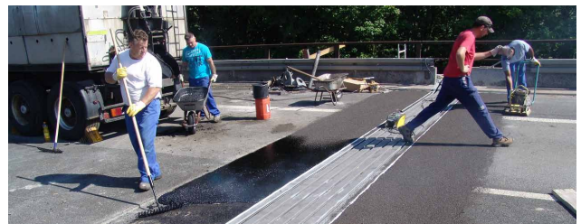
Restoration of sealing / surfacing
