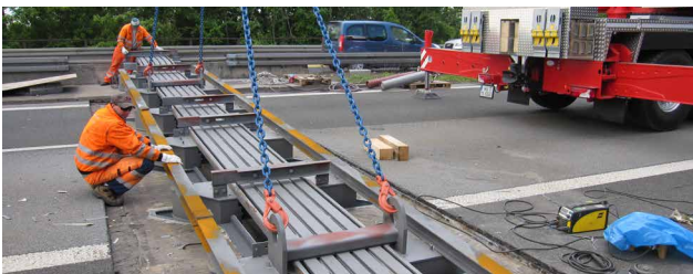
Lifting the new expansion joint into existing boxes
