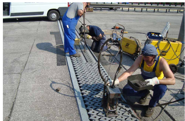
Welding of the rhombic elements with robot
