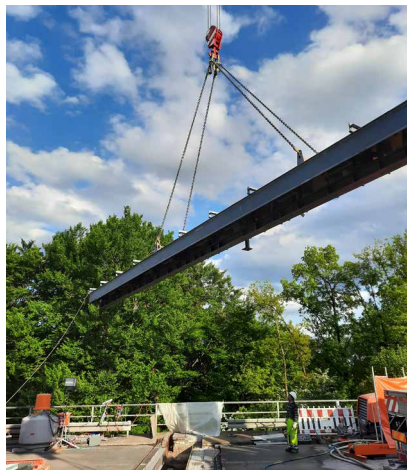
Lifting the new construction
