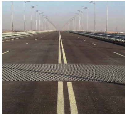
Noise reduction at swivel joist expansion joint
