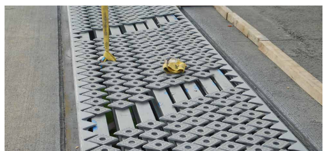
Installation of new centre beams with rhombic elements
