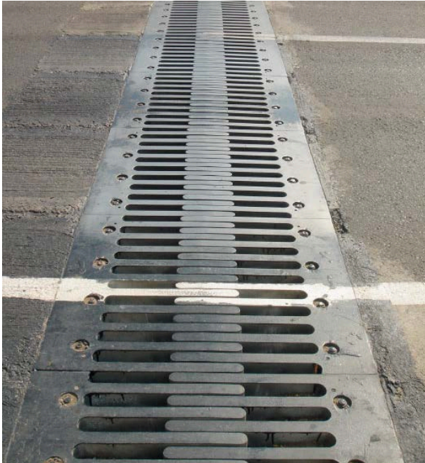
Fig. 1 – Finger joint
